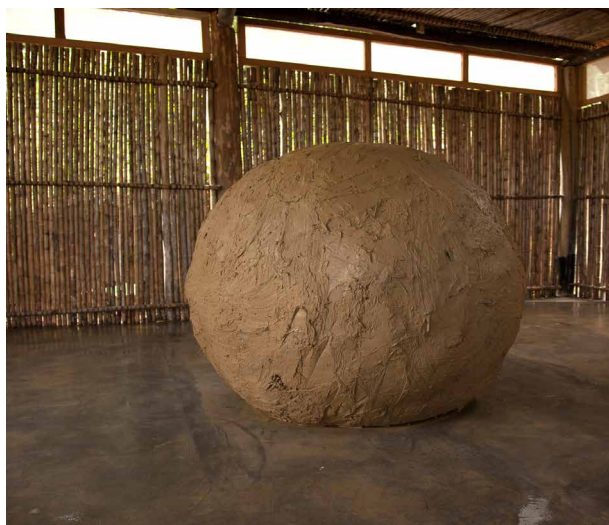
Fig. 5. Amazonico prototype recently plastered. The wet-mud skin is starting to collapse due the wobbling and vibrations. San Roque de Cumbaza, Peru. Summer 2013. Photo: Alejandro Borsani.
